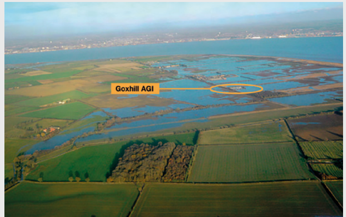
Figure 6.3: Flooding at the Goxhill above ground installation in 2013
