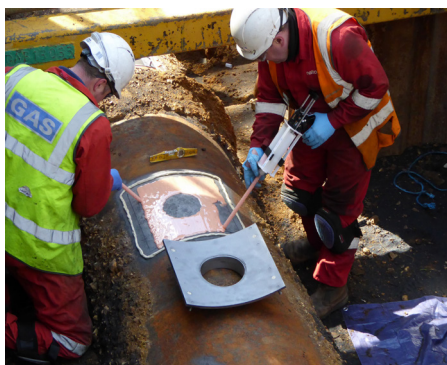
Applying the resin
