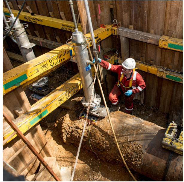
The pipe being cut out
