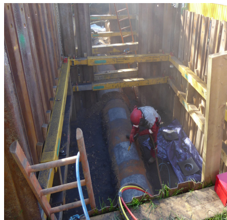
Shot-blasting the pipe
