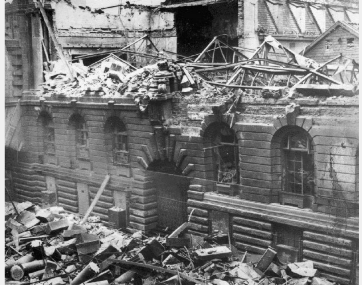
The Gas Department head offices after the air raids on the 21–22 November 1940. Source: National Grid Gas Archive
