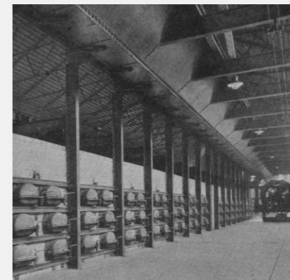
A view of the retorts and charging machine at Adderley Street Gasworks c1928. Source: National Grid Gas Archive.
