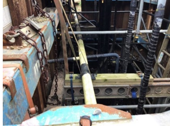
Figure 5: Temporary structure mitigating risk from clashing Actuator gas pipework movement
