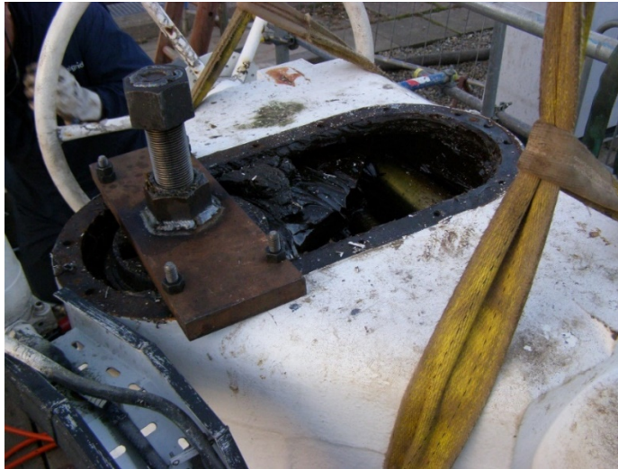
Figure 4 accessing valve 21074 for repair
