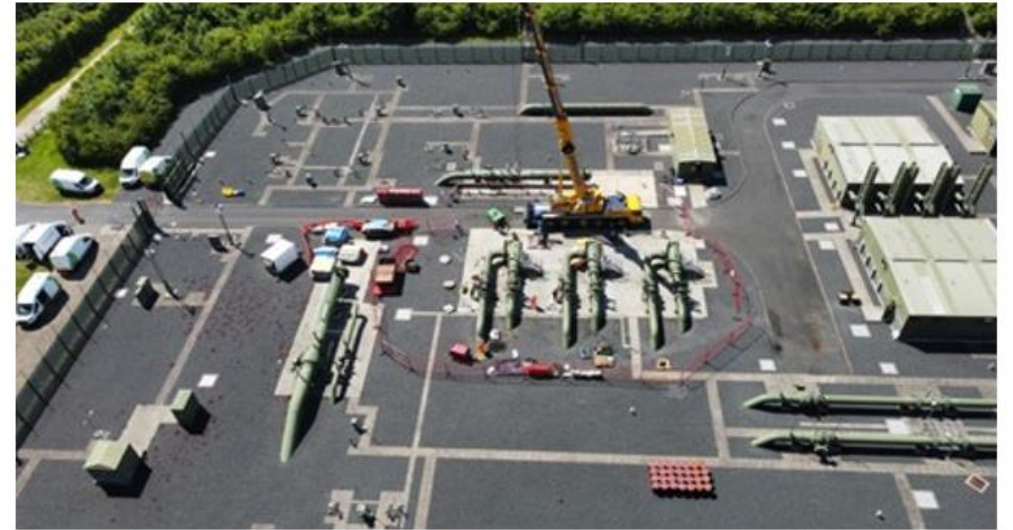
Construction work at Tirley PRI, June 2024
