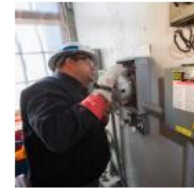
Unaccounted for Gas (UAG)
