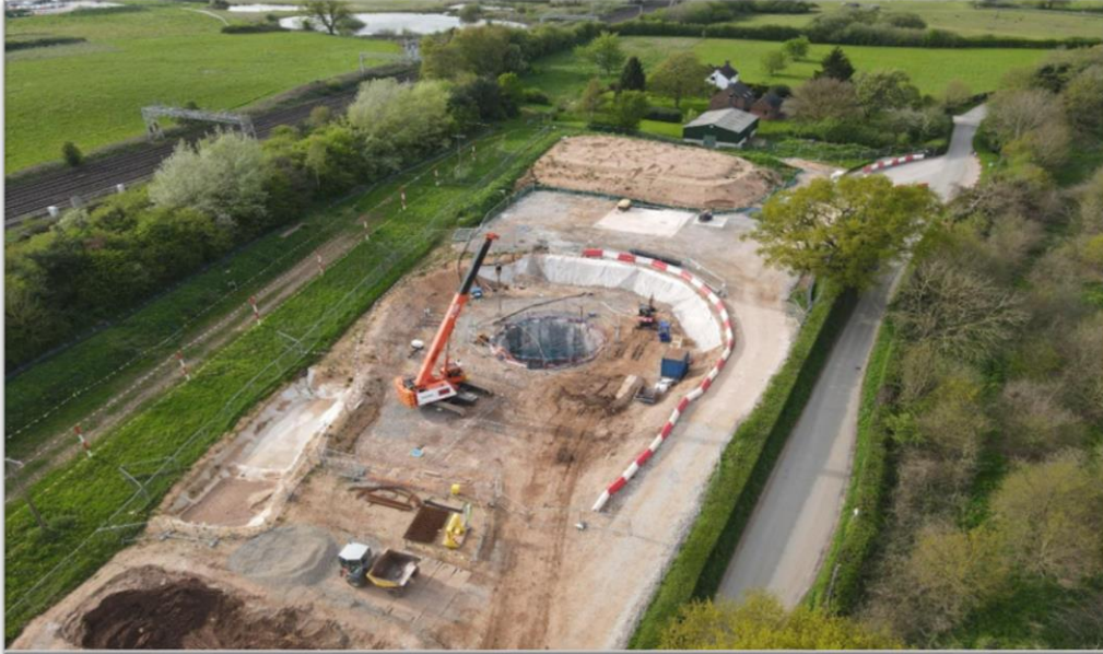
Figure 65 - TX35 launch shaft excavation works as of May 2023.
