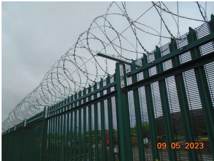
Figure 62 - Innovative fence retrofit fence upgrade solution at Barrington AGI
