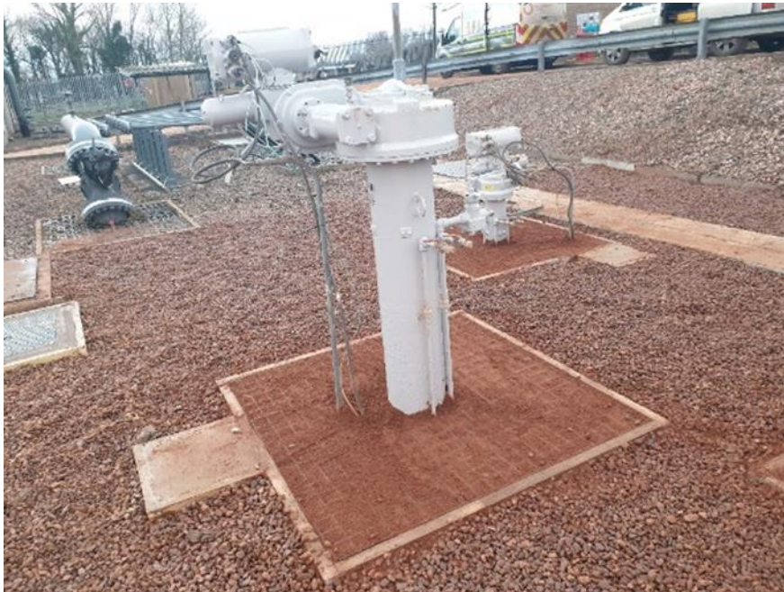
Figure 57 - Valves Refurbs – Aylesbeare Completion
