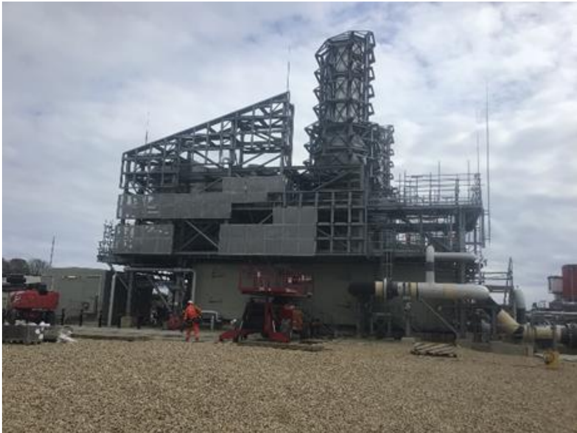
Figure 25 - New Compressor Unit cladding being fitted
