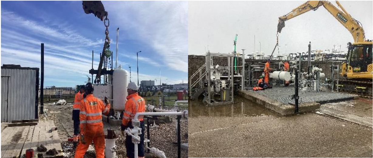
Figure 36 and 37 - Removal of old actuator and installation of new unit.
