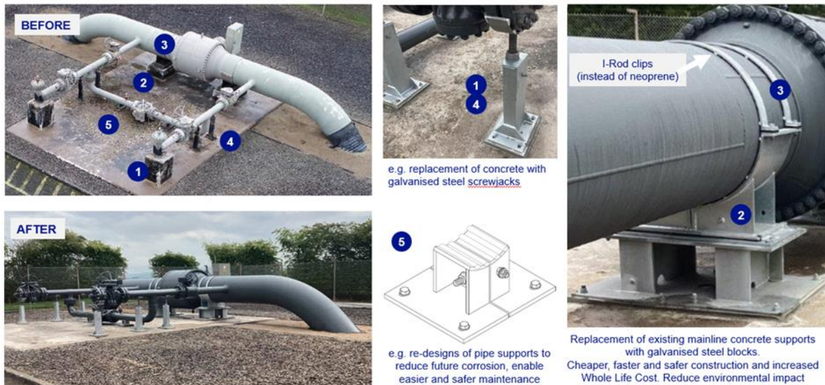
Figure 48 – Laurencekirk before and after implementation of pipe support innovations
