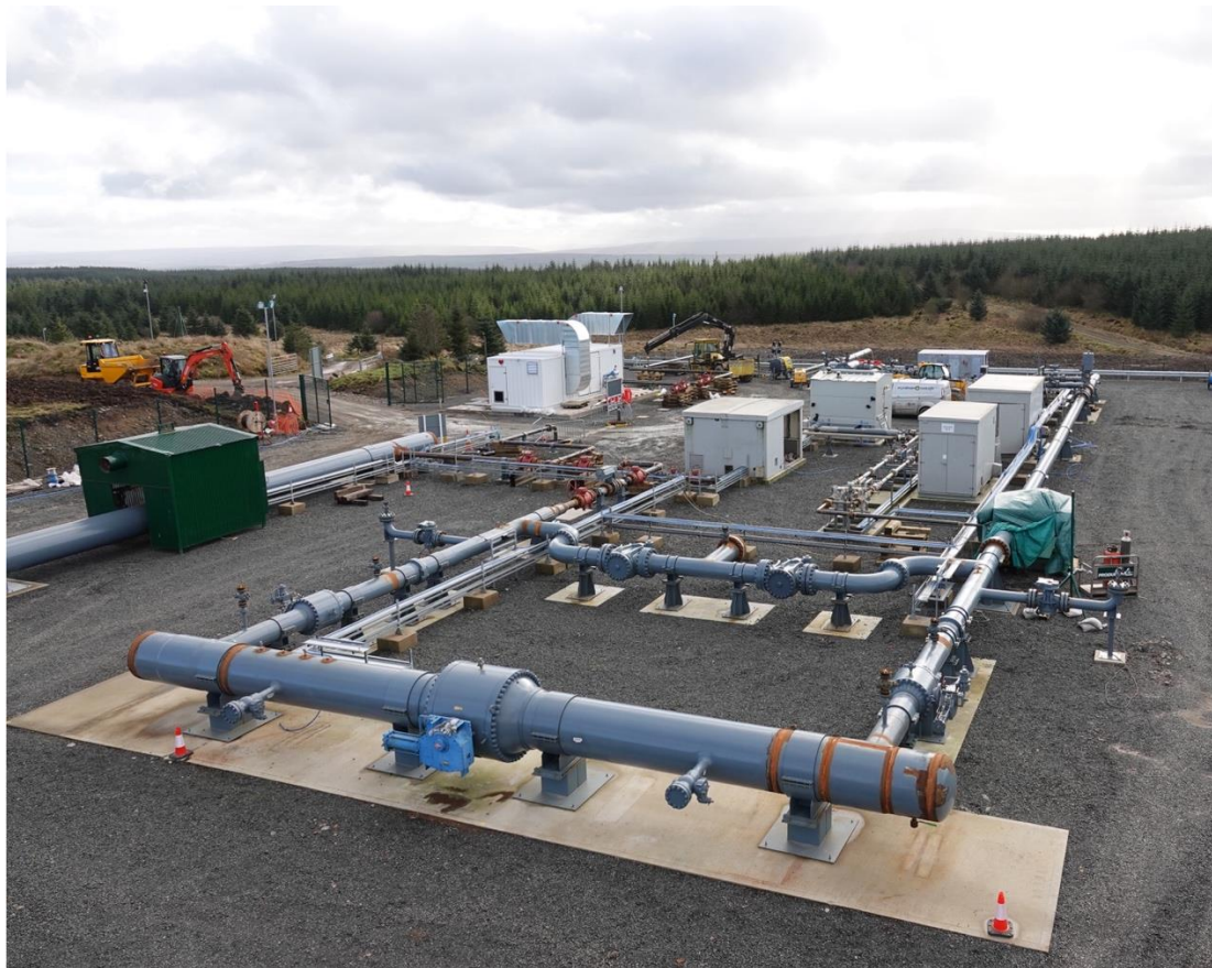
Figure 18 - FutureGrid Hydrogen Test Facility in final stages of construction in January 2023
