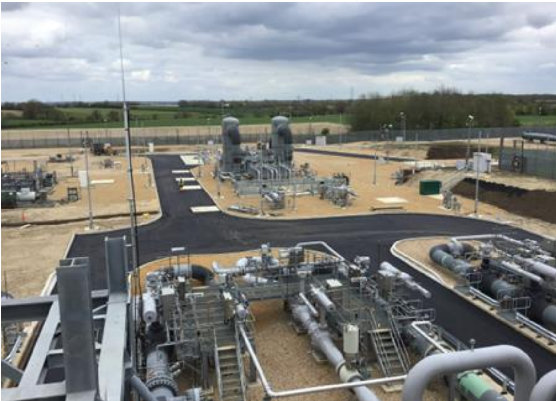
Figure 29 - Huntingdon site road finishing works
