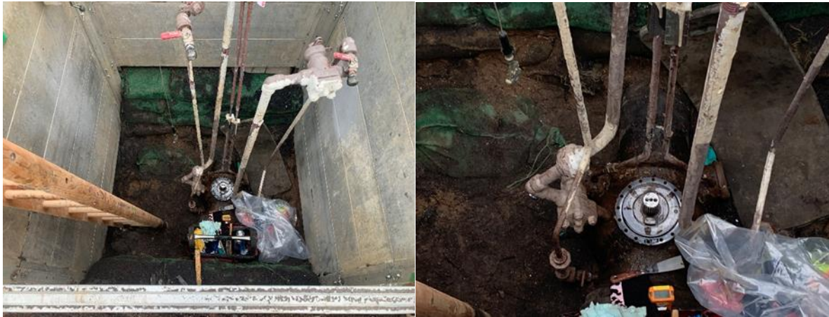
Figures 58 and 59 - Valve and spool replacement at Charlestown
