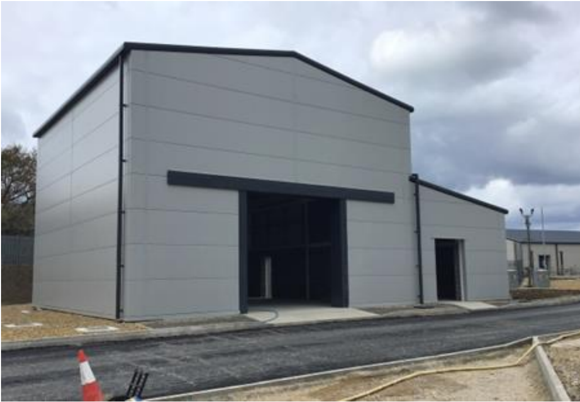
Figure 28 - New Maintenance Workshop at Huntingdon
