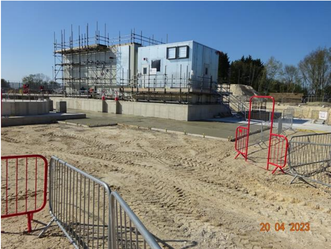
Figure 33 - New SGT-750 Compressor during installation
