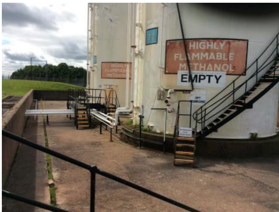
Figure 14 – St Fergus Methanol Tank (Pre decommissioning)
