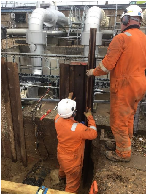
Figures 60 and 61 - Excavations underway at Bacton to facilitate buried pipework inspections
