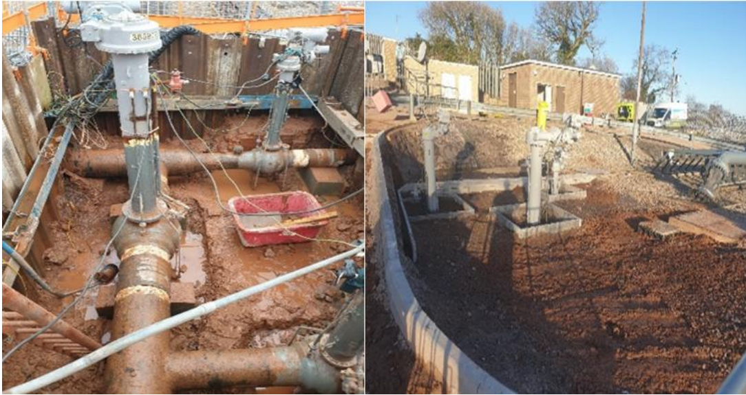
Figures 55 and 56 - Valves Refurbs – Aylesbeare During Construction
