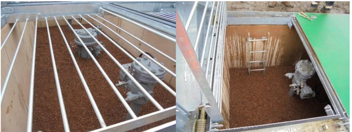
Figures 53 and 54 - Valves Refurbs Honiton – Completed/After
