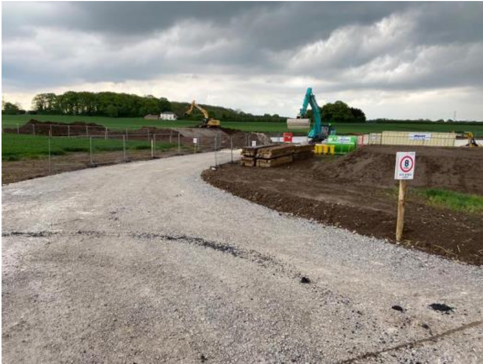
Figure 66 - Showing site establishing and ground works for A164 Diversion
