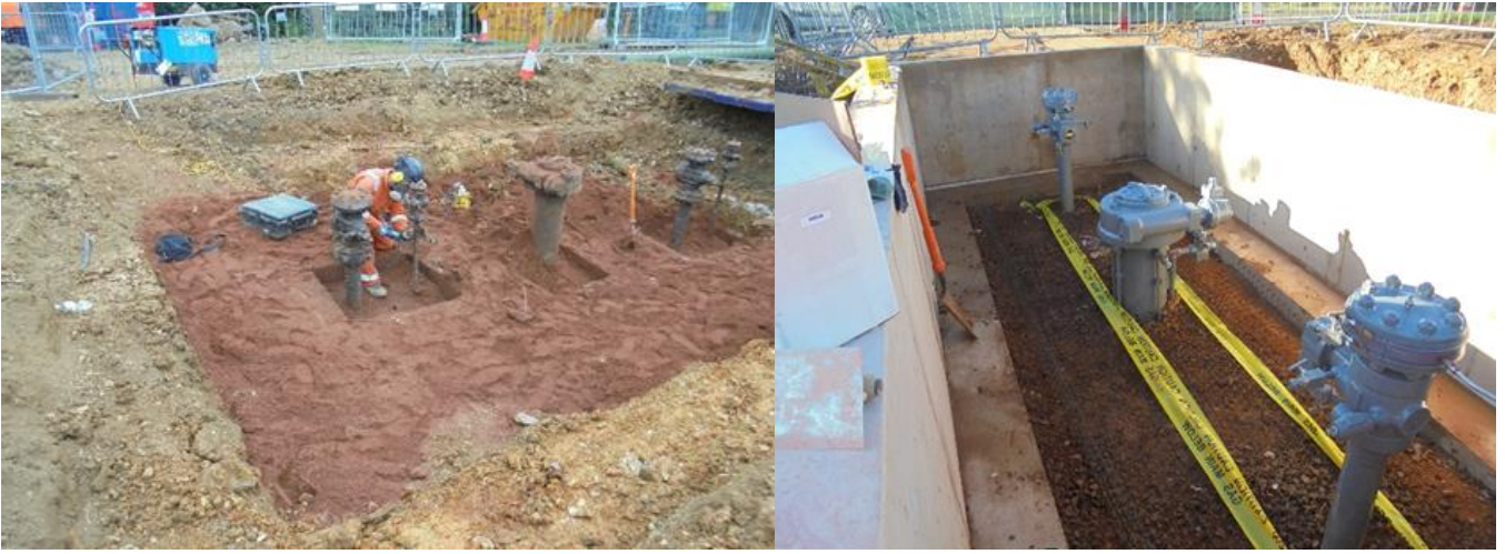
Figures 51 and 52 - Valves Refurbs Honiton – During Construction
