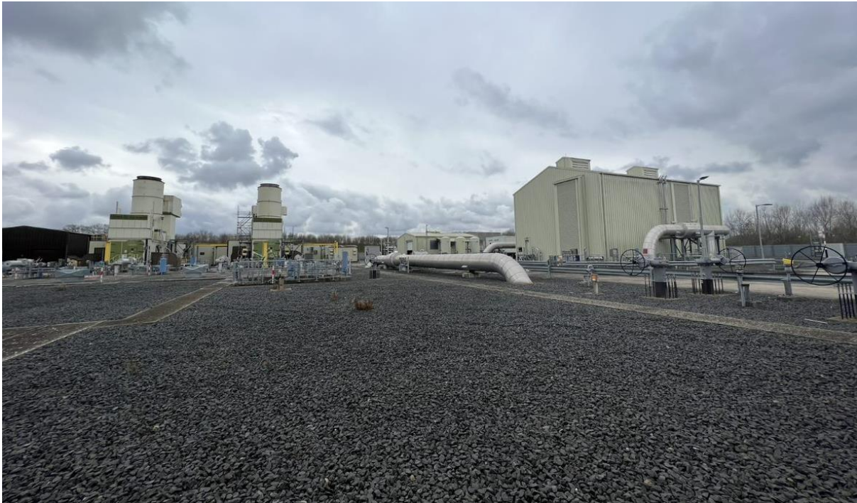
Figure 42 - Wormington Units A, B & C taken during site visit 7 March 2023
