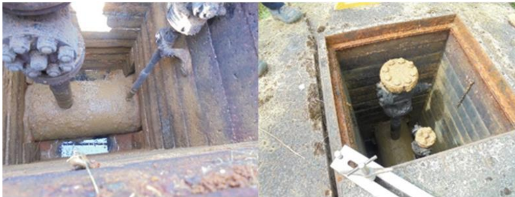
Figures 49 and 50 - Valves Refurbs Honiton – Pre-Construction
