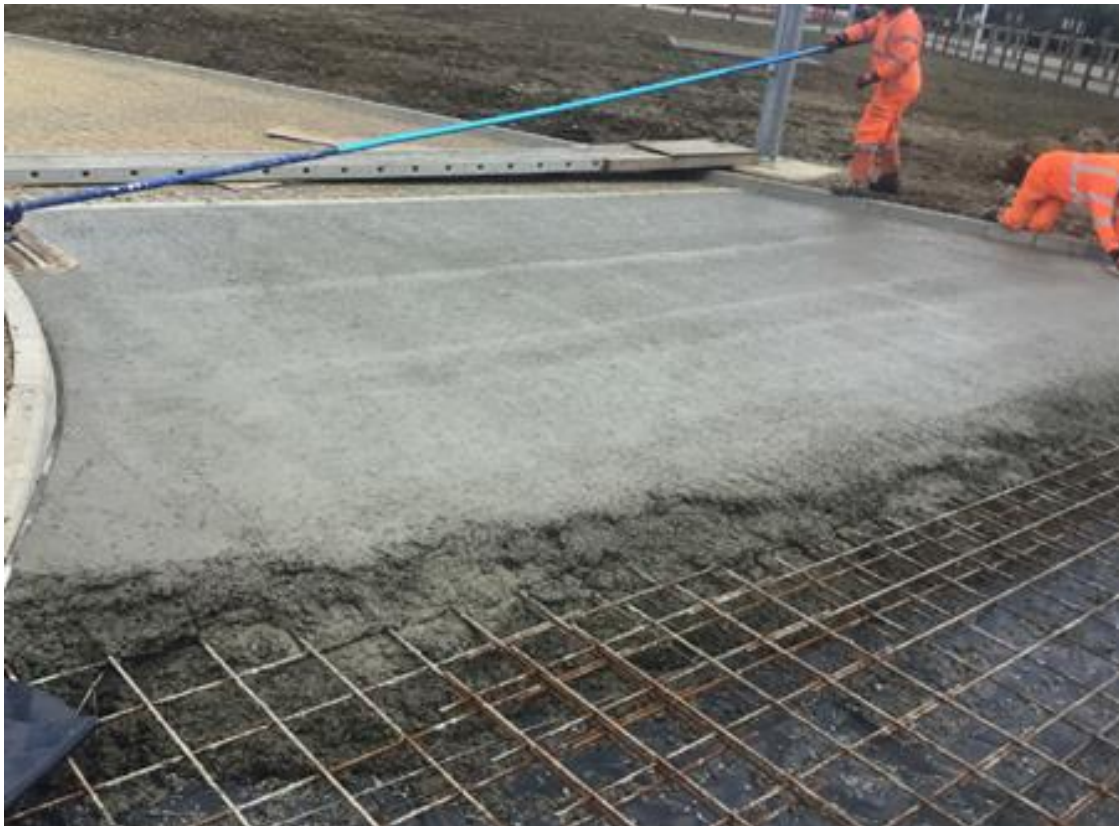
Figure 26 - Concrete being poured at Peterborough
