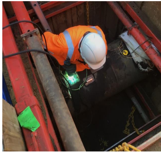
Figures 60 and 61 - Excavations underway at Bacton to facilitate buried pipework inspections
