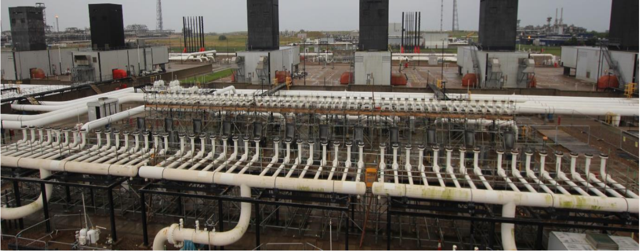
Figure 39 - Plant 1 following removal of aftercoolers
