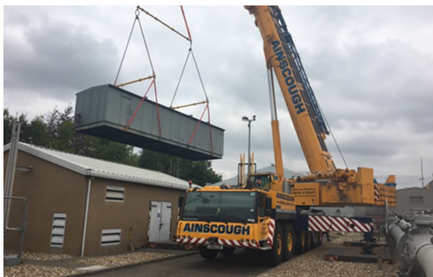
Figure 29 – The redundant boiler house being lifted out at Little Barford
