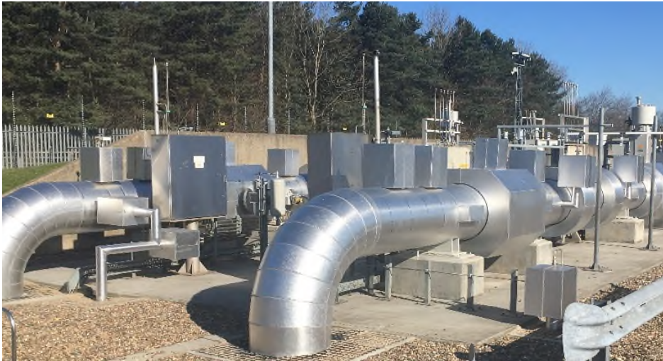
Figure 22: New acoustic cladding on Bishop Auckland regulator streams
