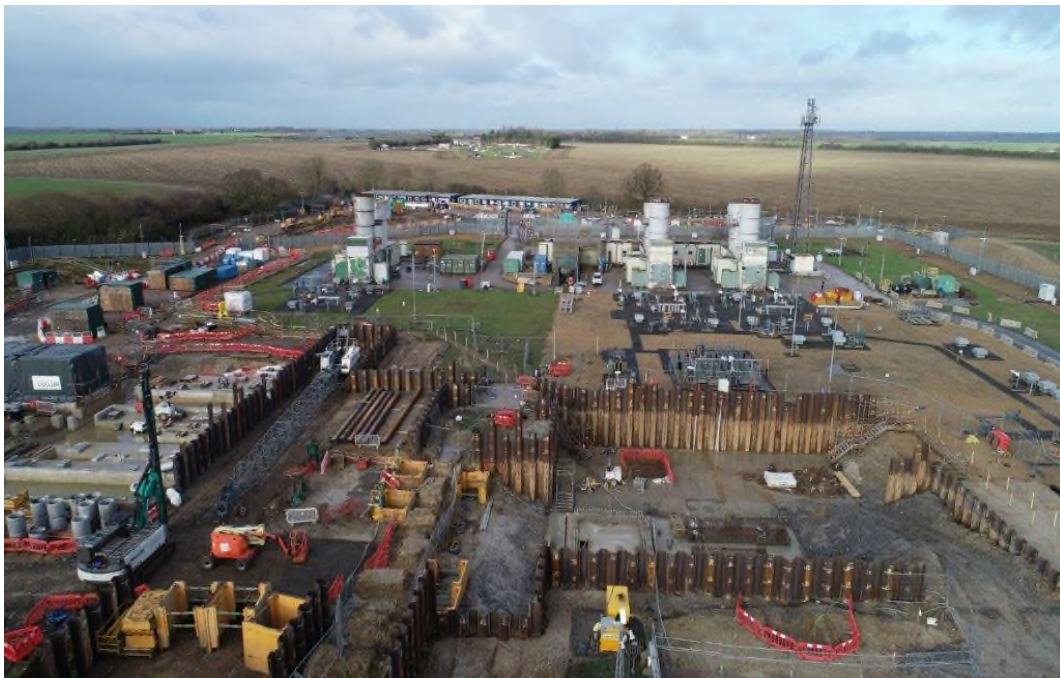
Figure 39: Ongoing Site Works at Huntingdon
