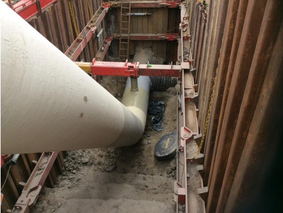
Figure 27: Installation of GRAID launch connection point
