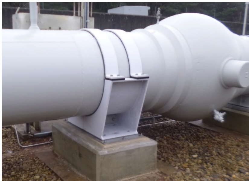
Figure 21: GRP pipe support installed at Bishop Auckland
