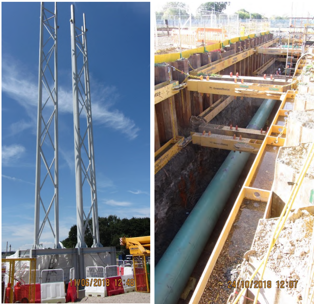
Figure 40: Ongoing Site Works at Peterborough
