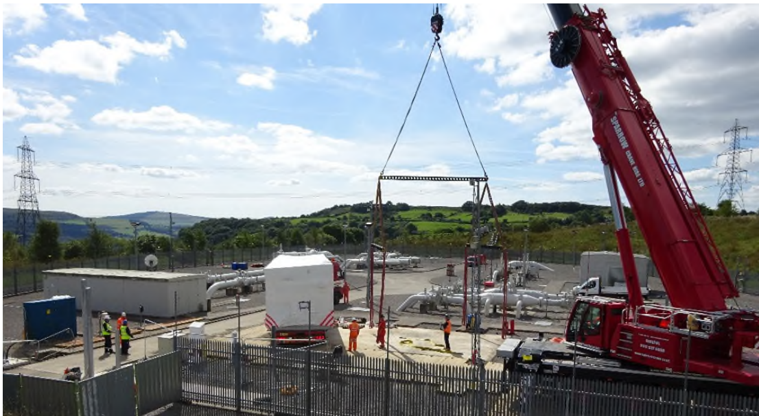
Figure 30 - Setting up of the Crane at Cilfrew
