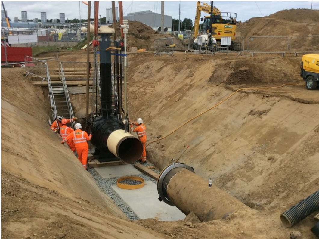
Figure 25: Installation of new isolation valve (Phase 3a)
