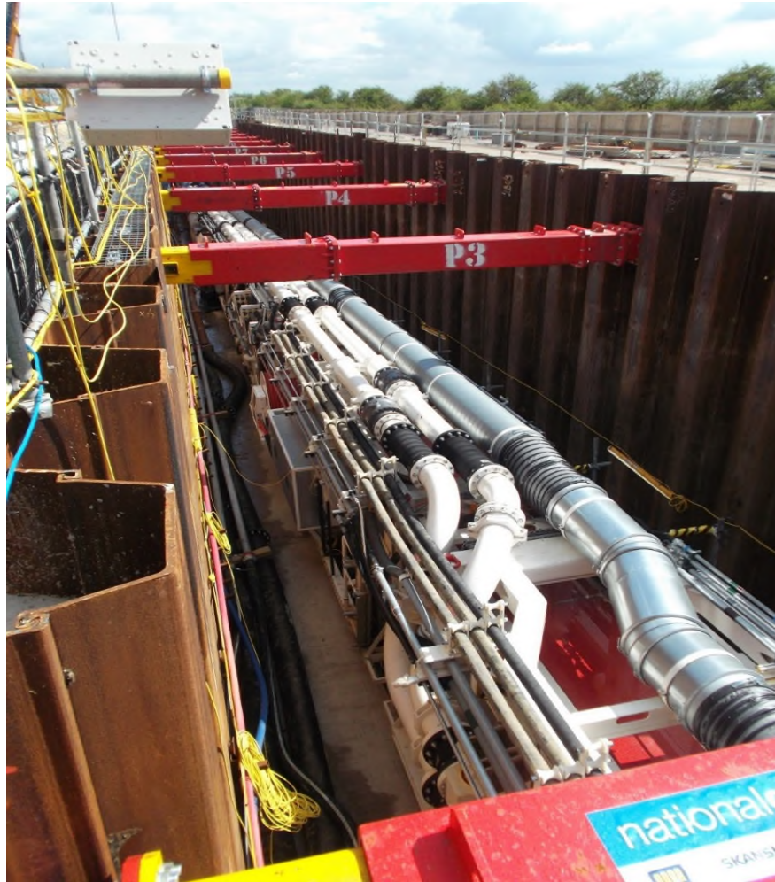
Construction of reception shaft at Paull
