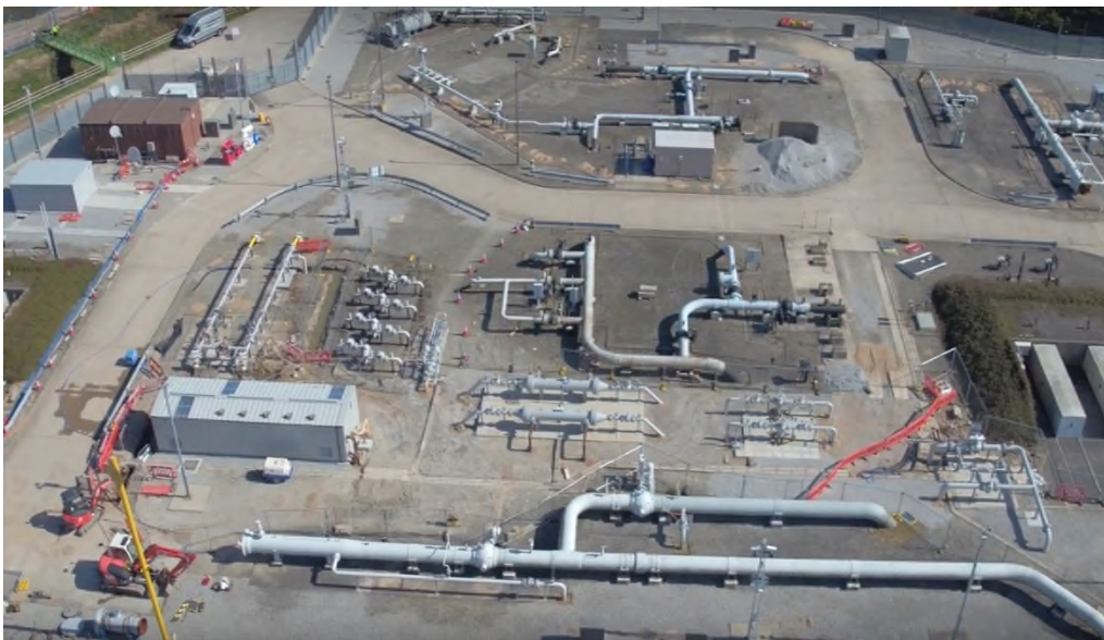
Figure 36: Paull site equipment post rationalisation (2018)
