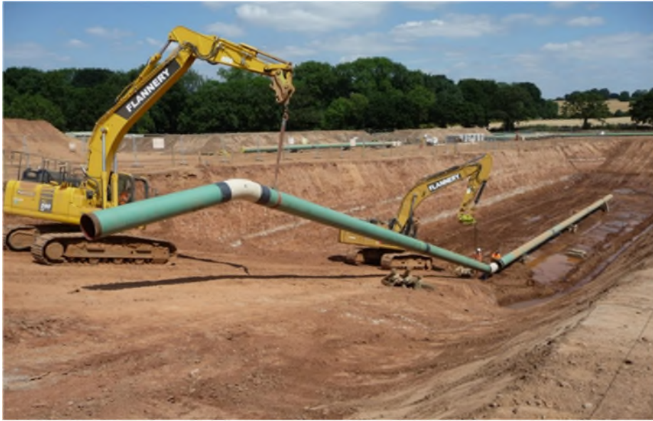
Figure 42 and 43 - Pipeline being installed into a cutting as part of the TX05 Diversion
