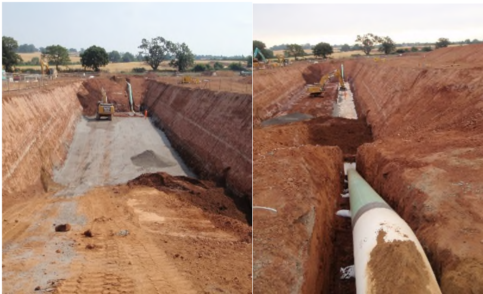
Figure 42 and 43 - Pipeline being installed into a cutting as part of the TX05 Diversion
