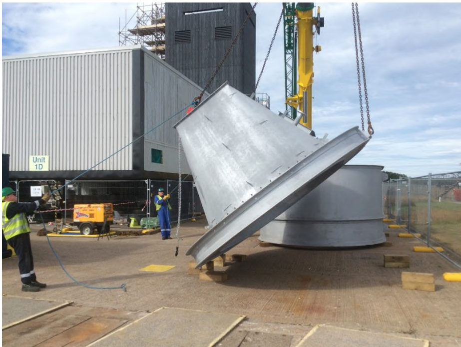
Figure 24 – Installation of replacement exhaust (bottom section) Cab 1D St Fergus
