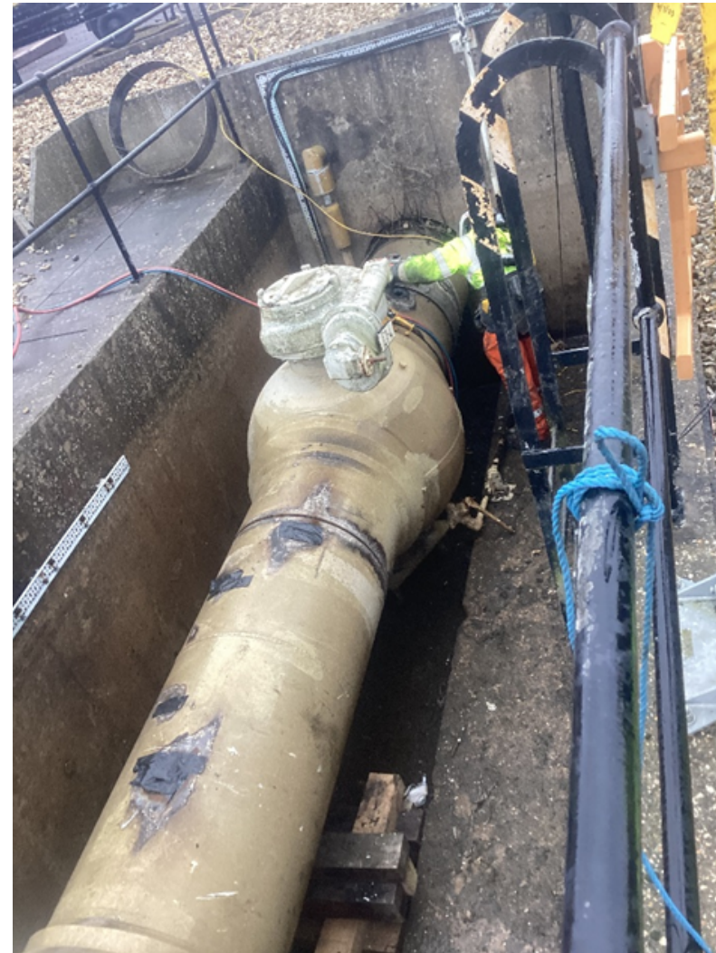
Figure 13 - An uncovered valve due for decommissioning at Theddlethorpe
