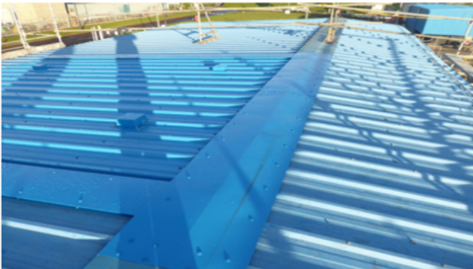
Hatch installed – all works complete
