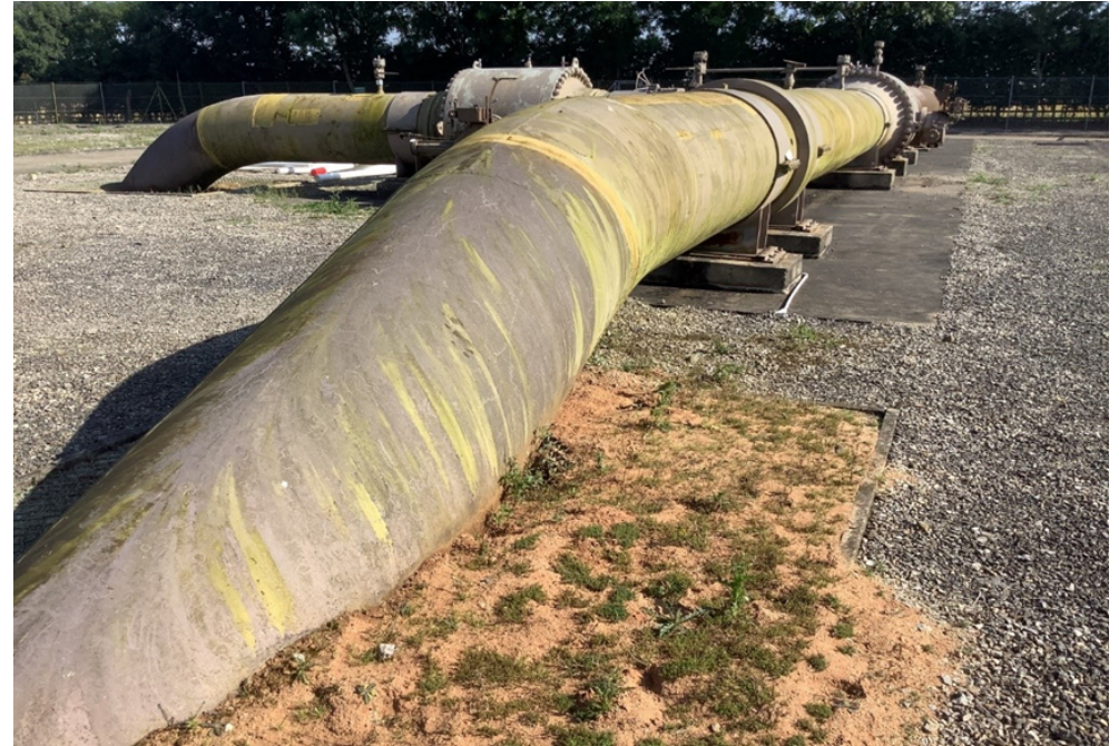
Figure 38 – Site condition photos before asset health works commenced
