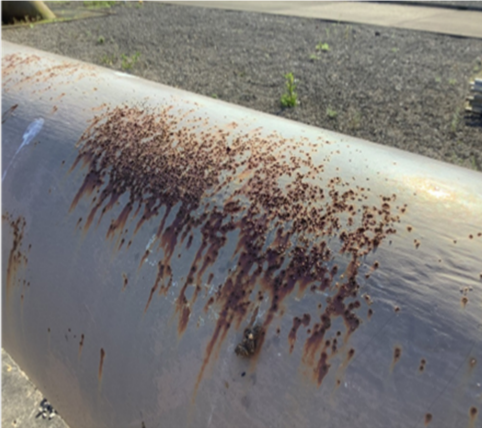
Figures 37 – Site condition photos before asset health works commenced
