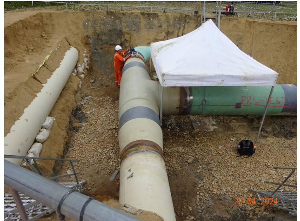
Figure 27 - Tie ins being completed
