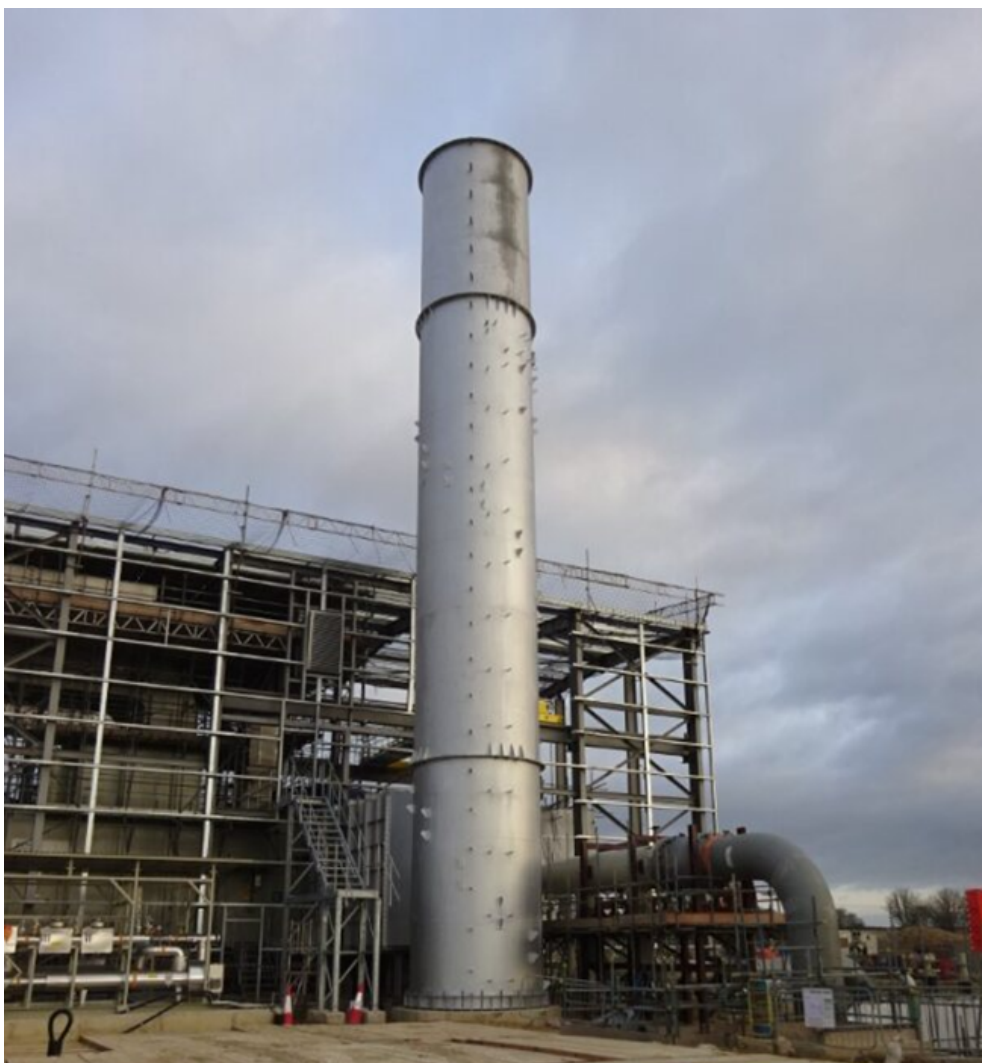
Figure 28 - Exhaust stack erected around the GT compressor
