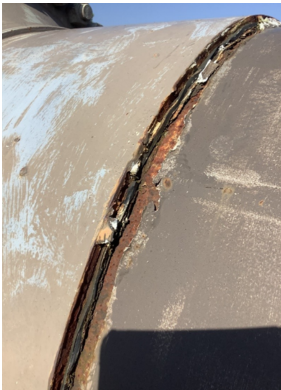
Figure 39 - Site condition photos before asset health works commenced
