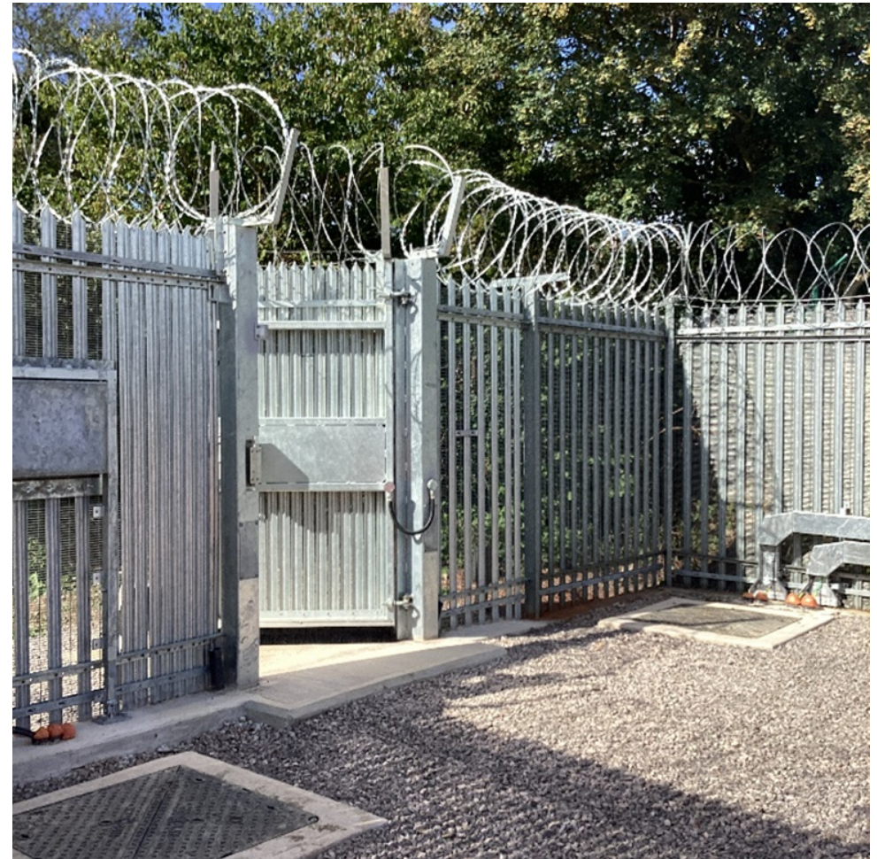
Figure 60 – Fencing and pedestrian gate
