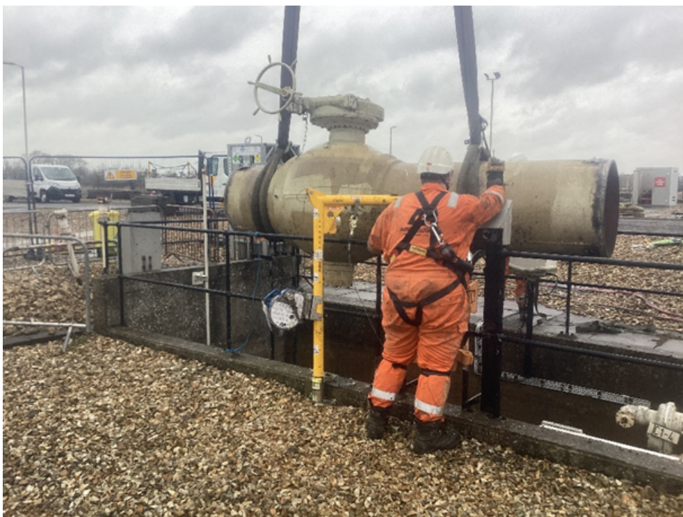
Figure 14 - Crane valve removal at Theddlethorpe
