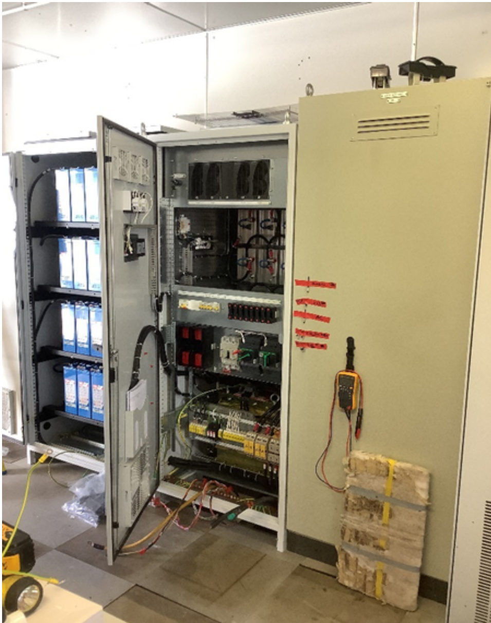
Figure 49 - New batteries and charger system installation at Wooler Compressor
