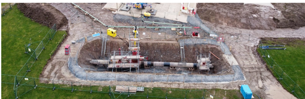
Figure 58 - Lockerbie Stopple intervention
