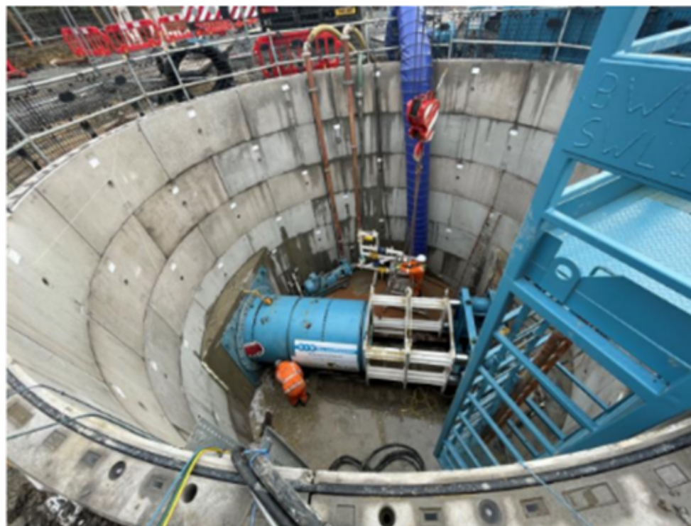
Figure 62 - Micro tunnelling at the A47 National Highways project
