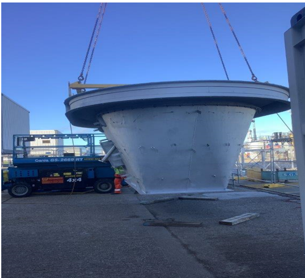
Figure 33 – Cab 2B GT exhaust transition piece after re-life
