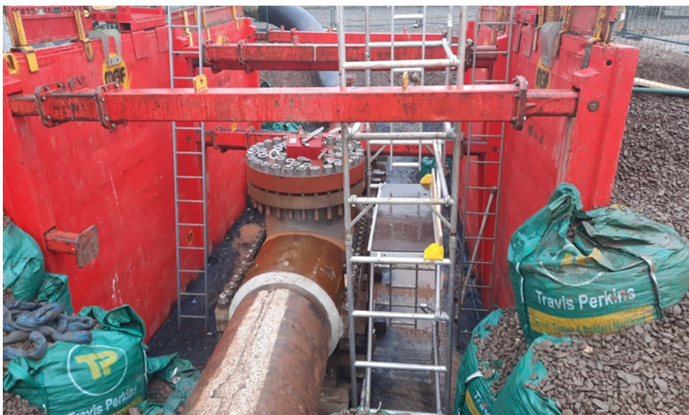
Figure 57 - Longtown Stopple intervention
