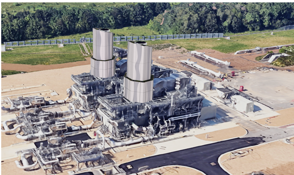
Figure 23 - Design for exhaust stack cladding at Peterborough
