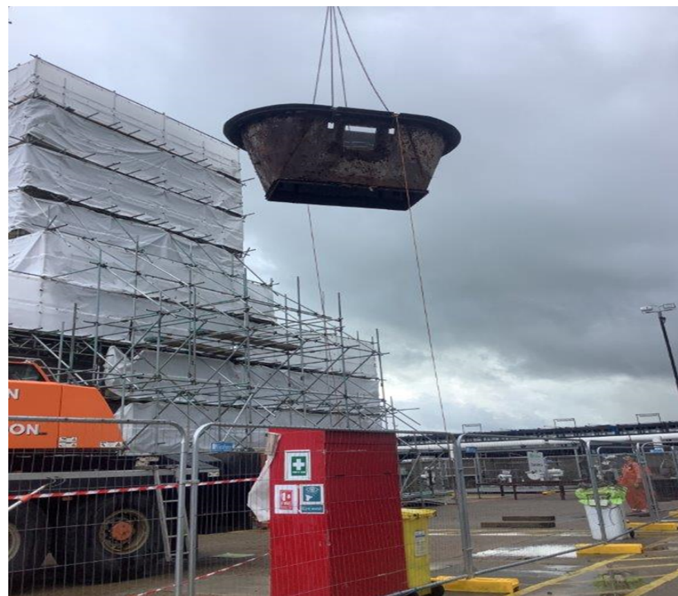
Figure 32 - Cab 2B GT exhaust transition piece before re-life
