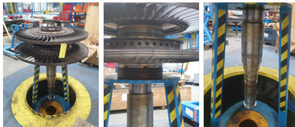
Figure 45 – Huntingdon Unit C: RT48S on Receipt Inspection
