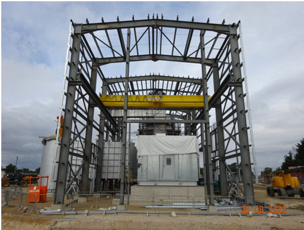
Figure 26 - Steel work to form the noise attenuation
