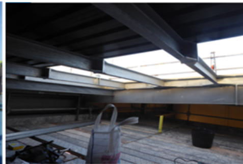
Roof prepared for new hatch to be installed
