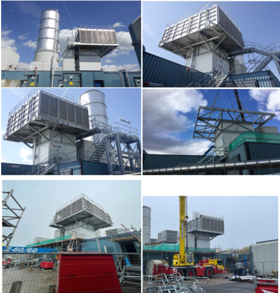
Figure 52 - Air intake filter house and exhaust works
