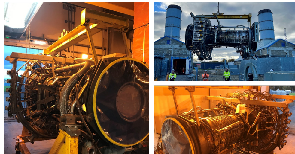
Figure 43 – Engine exchange at Bishop Auckland.
