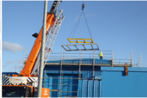
Hatch being lifted into position
