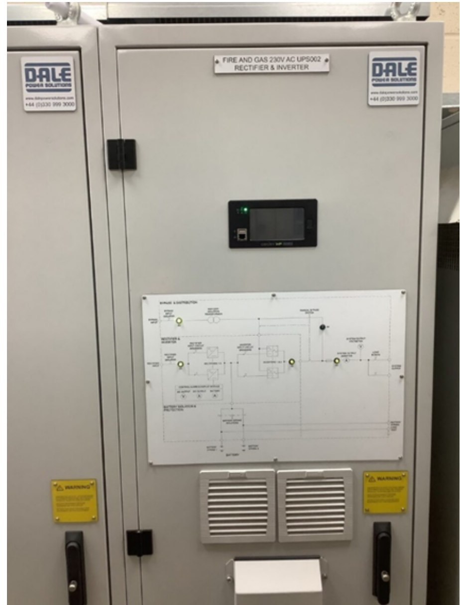
Figure 50 - Replacement Fire/Gas uninterruptible power supply at Nether Kellett Compressor.
