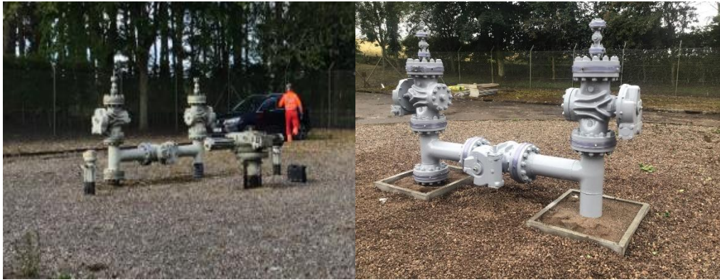
Figure 32 and 33: Before and after photos of Milnathort Block Valve site
