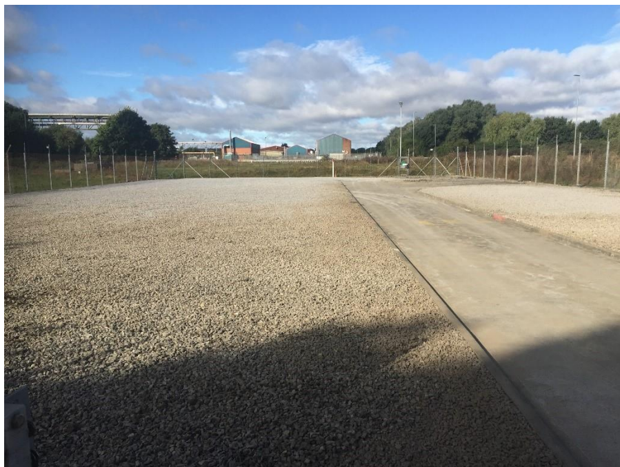
Figure 10: Demolition works on site at Enron Billingham AGI
