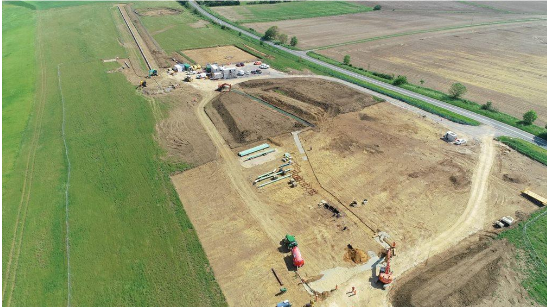
Figure 42: A428 diversion arial view– pipeline string ready for directional drill pull
