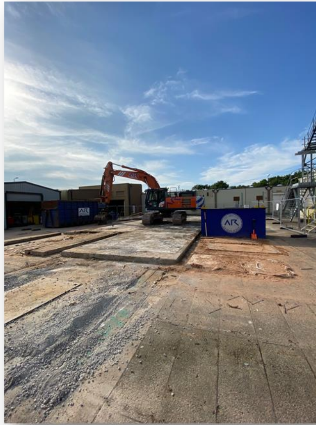
Figure 9: Demolition works on site at Carnforth (Unit A)
