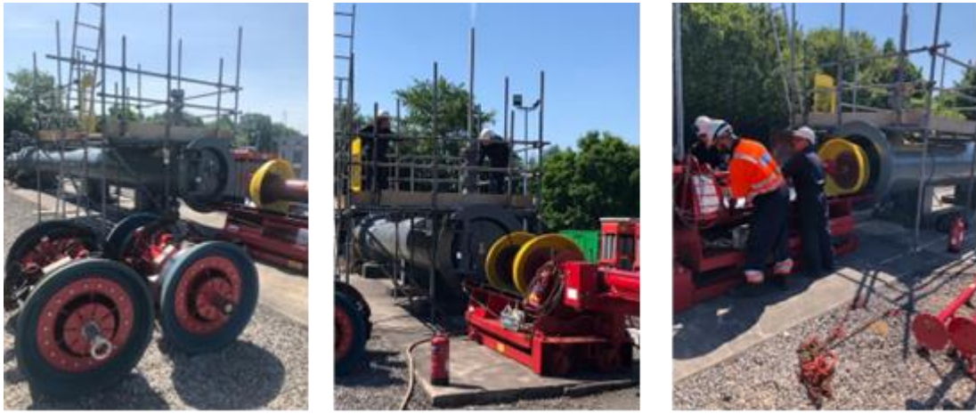
Figure 36: In line Inspections (using various PIGs) underway
