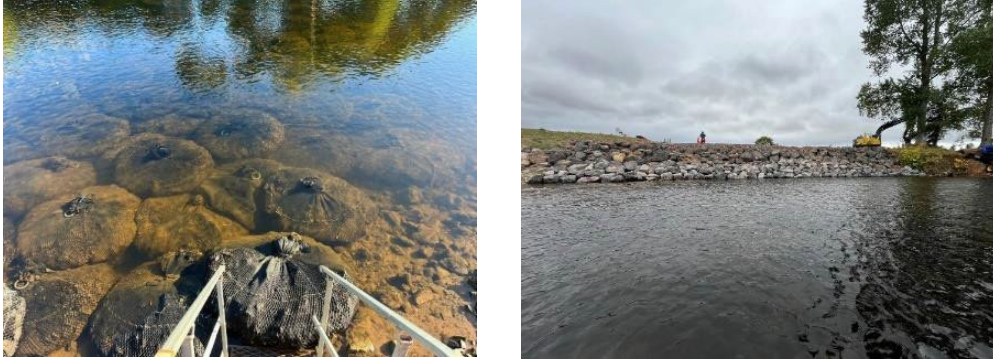
Figure 6 (left) Rock bags to reinstate DOC [REDACTED]
