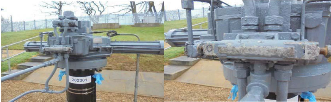
Figure 3: Defective [REDACTED] Gas-Hydraulic actuator
