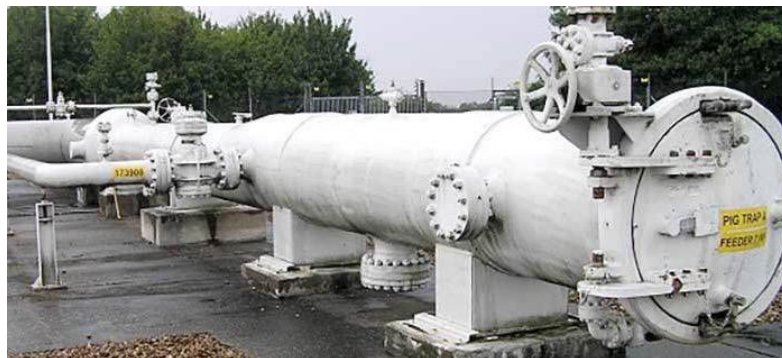
Figure 2: PIG Trap A on Feeder 7
