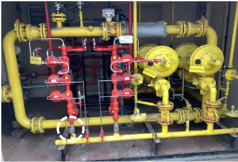
Figure 6 Stream A and B slamshuts (circled) with the bypass lines at [redacted]
