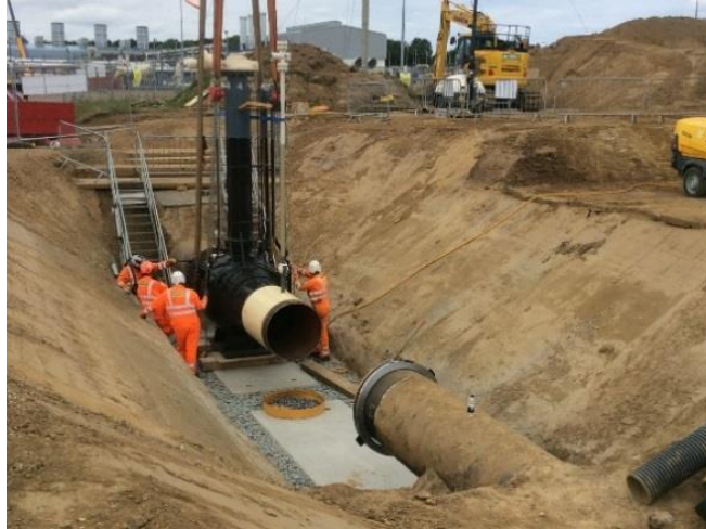
Figure 10: Example of valve replacement work
