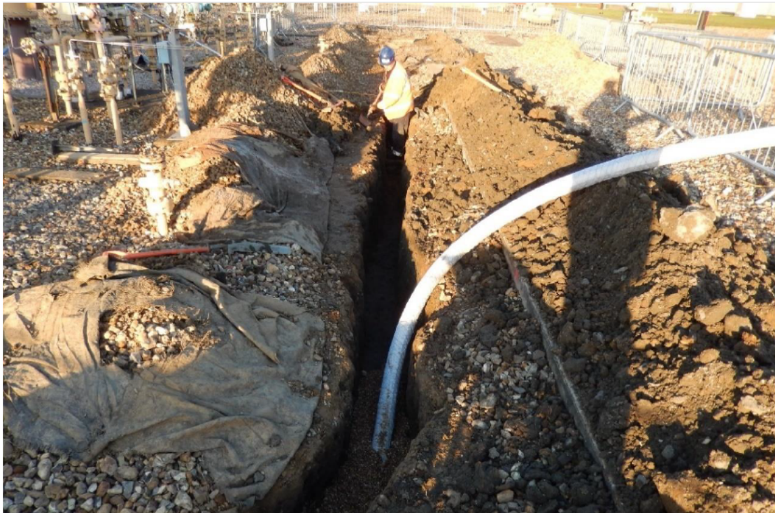
Photo 2 Installation of land drain (Winter 18/19)
