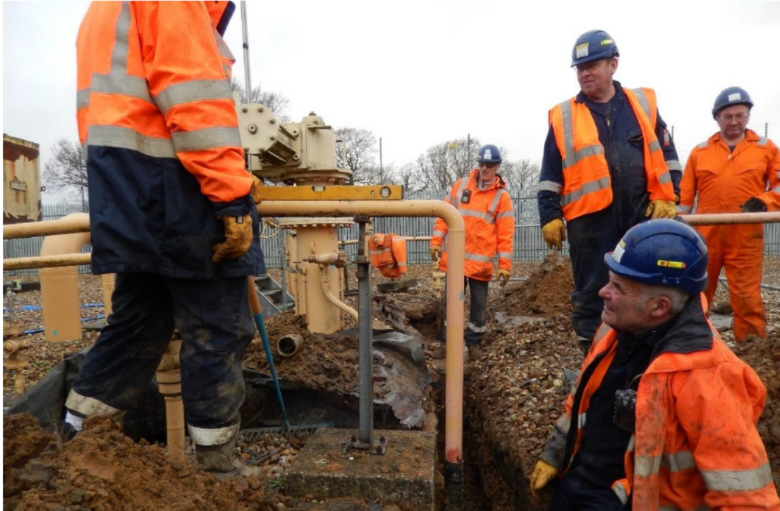
Photo 1 Excavation of 50NB pipework, stress relieving & re-levelling (Winter 18/19)
