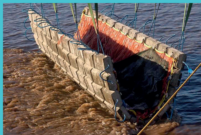
Concrete mattresses used to protect the existing Feeder 9 pipeline
