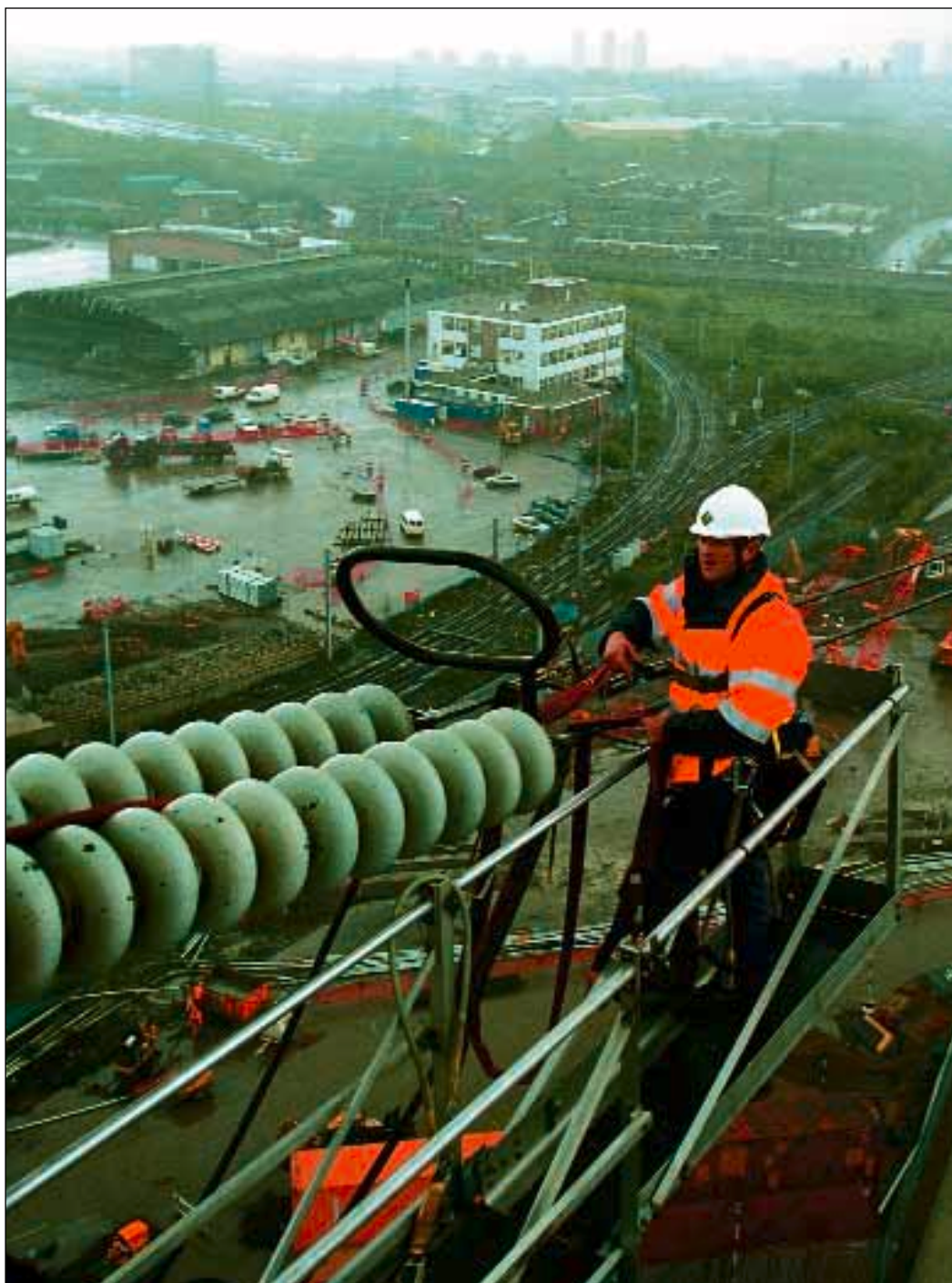
Overhead line refurbishment work near Hackney Marshes, north east London
