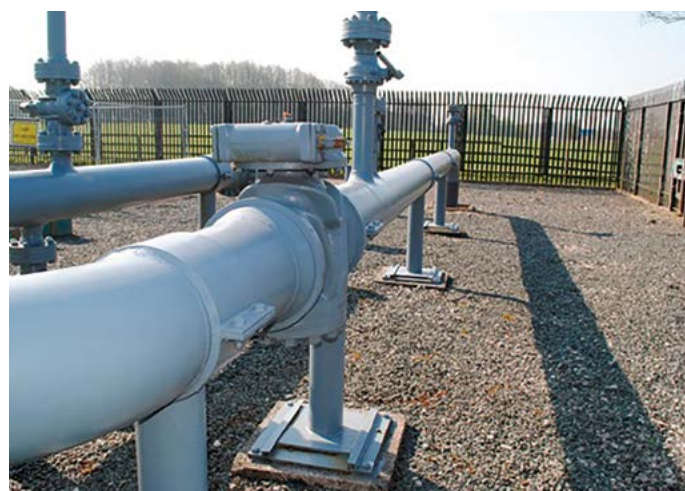
Refurbishment of site pipework on HP reduction installation.
