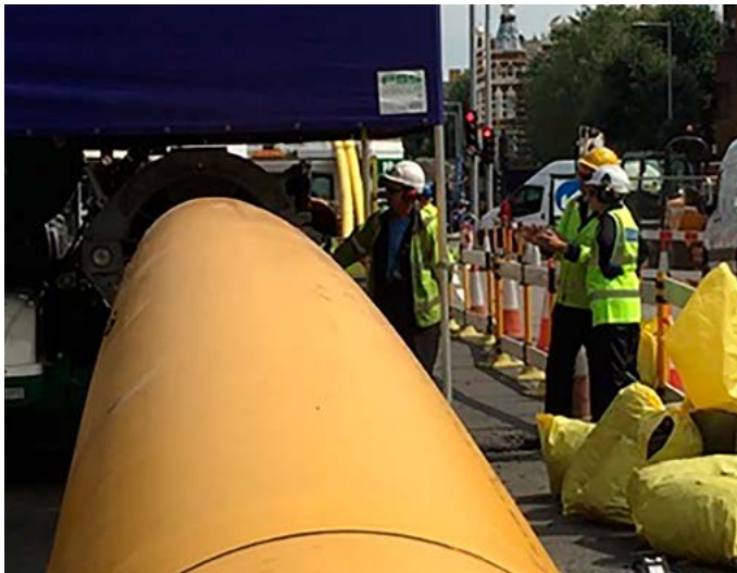
Replacement of metallic pipeline, Kings Road, London
