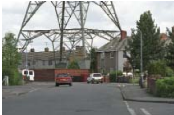
How not to approach the siting of homes near overhead power lines.
