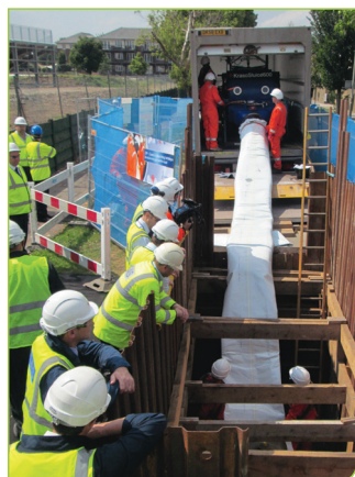
The CIPP technique being monitored by engineers.
