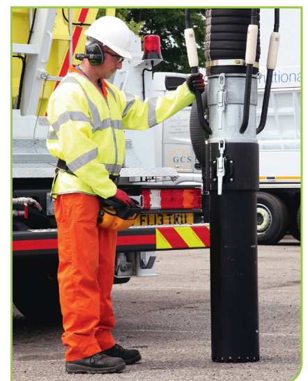
The Core and Vac process taking place.
