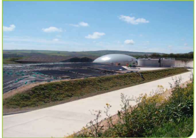
Poundbury, the UK's first full-scale anaerobic digester and biomethane-to-grid plant.
