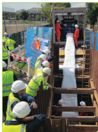
The CIPP technique being monitored by engineers.
