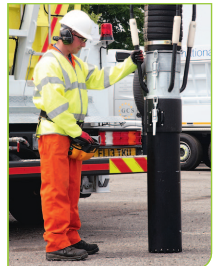
The Core and Vac process taking place.
