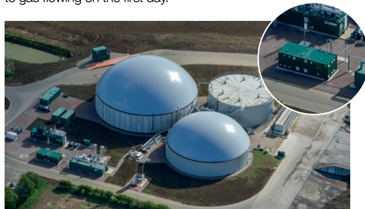
Bio-methane installation with single box grid entry unit Inset: Single box grid entry unit
