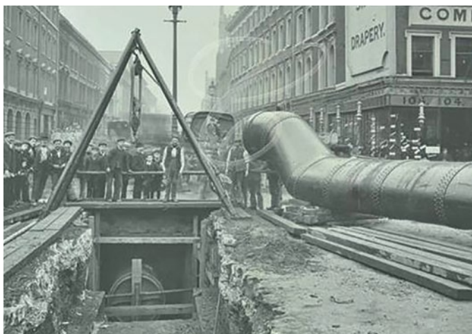
Victorian metallic pipeline
