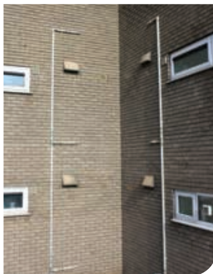
Below and Right: Vertical Polyethylene (PE) risers to three-storey flats at Walsall Housing Group
