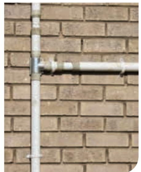
Below and Right: Vertical Polyethylene (PE) risers to three-storey flats at Walsall Housing Group
