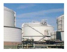
LNG tanks are always of double-wall construction with extremely efficient insulation between the walls. Large tanks generally have a low aspect ratio (height to width) and are cylindrical in design with a domed roof. Storage pressures in these tanks are very low, less than 120mb. Smaller quantities tend to be stored in vacuum-jacketed, pressure vessels. These tanks may operate at pressures from a few millibars to 18 barg.
