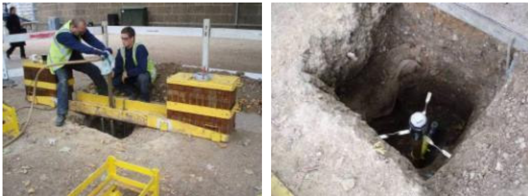
Typical excavation required to drill tap and install pressure & bypass points on 48" Main Using the Beam Drilling System
