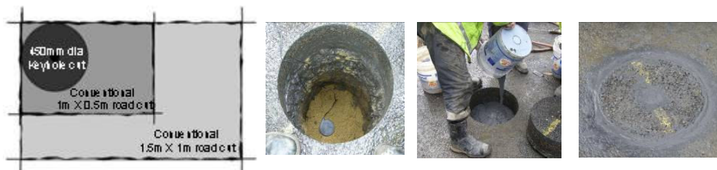
Figure a2.3 - Illustration of Keyhole technology repair process
