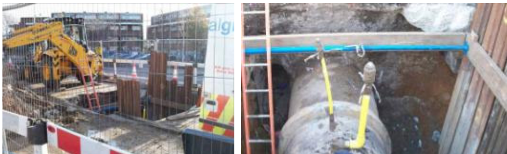
Typical excavation required to drill tap and install pressure & bypass points on 48" Main. Excavation required enabling a chain to be passed under the main to secure the drilling base
