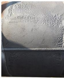
The photos above show the pipe support prior to the works being commenced and an example of the type of corrosion that was found on the pipe.
