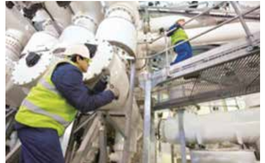
Sulphur Hexafluoride Leak Management
