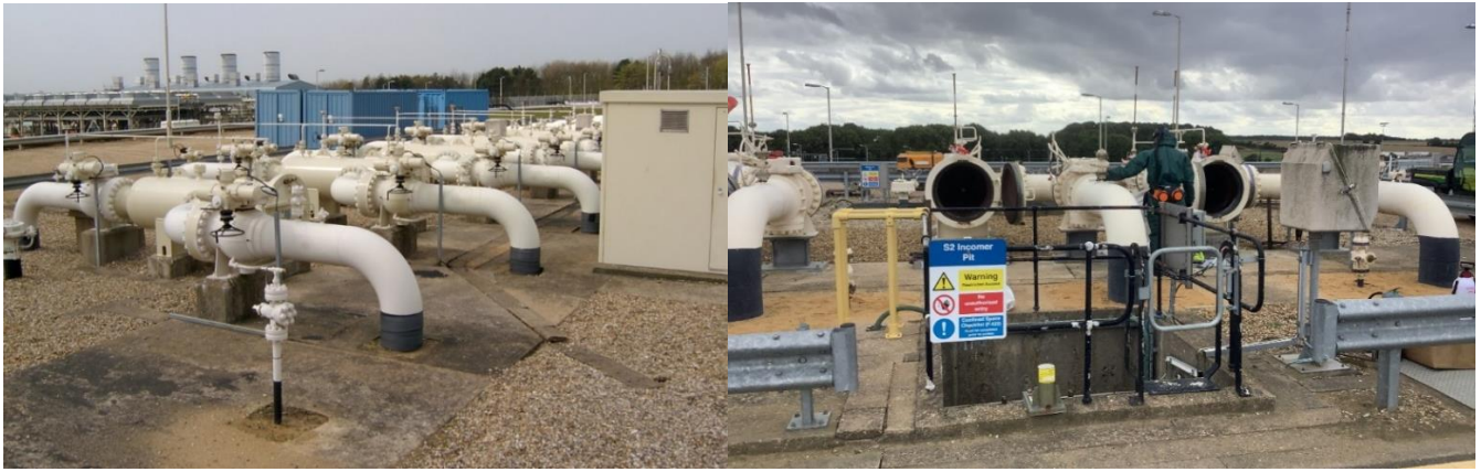
Figure 22: Class 600 Horizontal Filter Vessel
